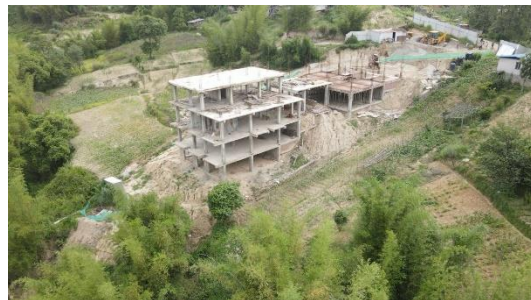
Hospice Building under construction
